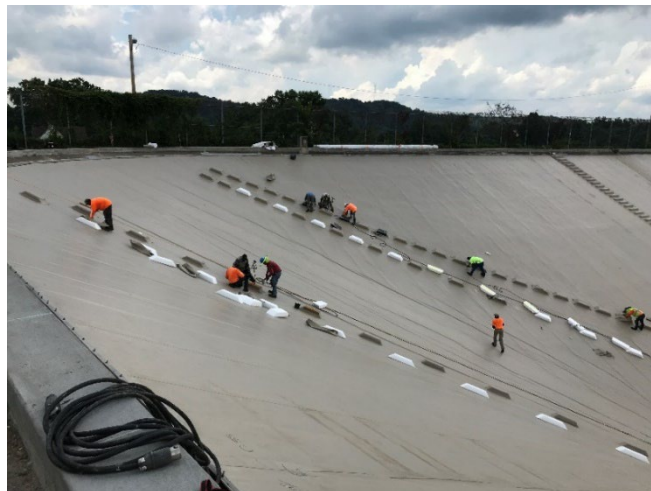
Figure 7. Crew installing floats and caps near Pittsburgh, PA.
