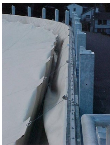
Figure 5. Tension cable and towers
