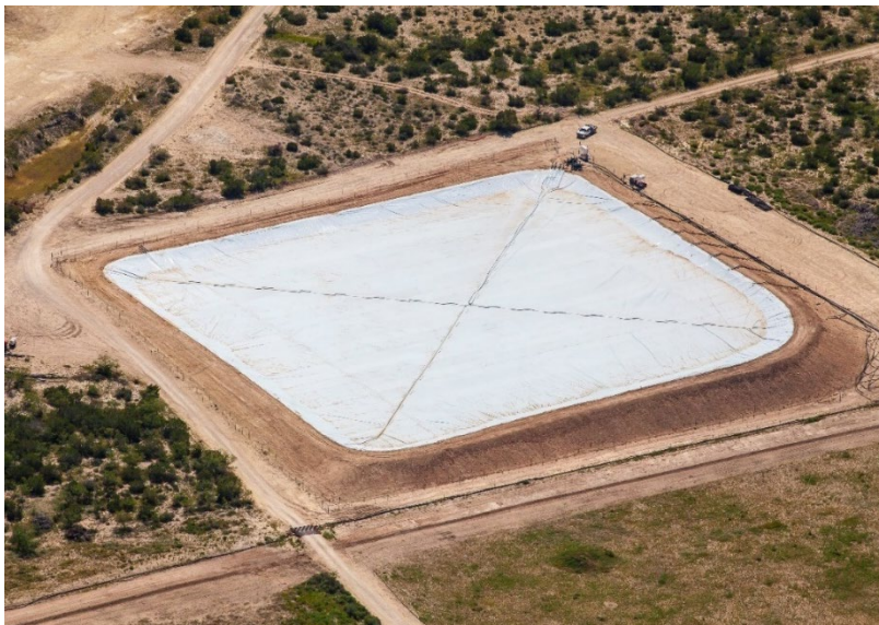
Figure 2. Evaporation control floating cover, West Texas, USA
