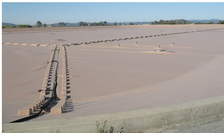
Figure 3. Defined sump cover in operation
