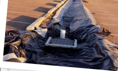
Also known as infiltration swales, Bioswales are a form of bioretention designed to slow surface water runoff and help in the removal of stormwater pollutants. Unlike ditches, they slow down the movement of runoff allowing the water to be cleaned and filtered along the way. Bioswales can be used in many applications including pollutant removal, drainage retrofitting, and runoff management.
