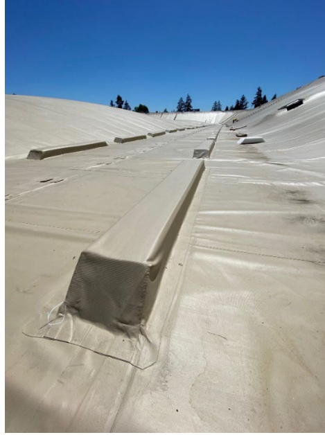
Figure 7 and 8. Inflation via access hatch and west cell cover undergoing inflation inspections.
