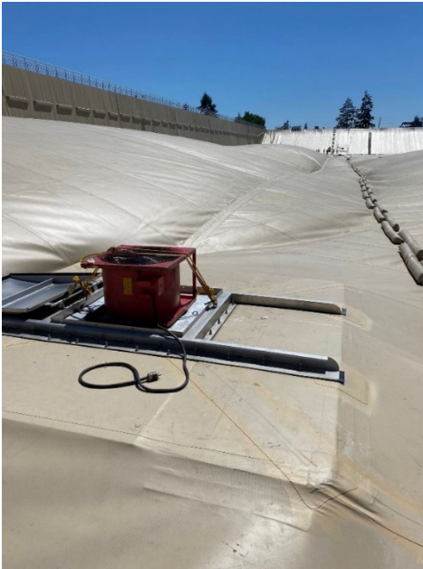
Figure 7 and 8. Inflation via access hatch and west cell cover undergoing inflation inspections.
