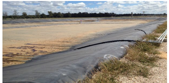
Figure 6. 1.00mm proprietary polyolefin floating cover on syngas process water to eliminate odors and rainfall ingress. Qld, Australia (Image: A. Gersch, 2015)
