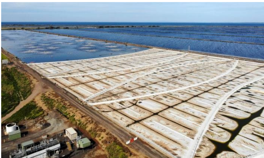
Figure 2. HDPE Floating cover on the anaerobic section of a wastewater treatment lagoon capturing biogas and eliminating odors. An energy company has an offtake agreement with the municipal water authority to use the gas to generate electricity. Victoria, Australia. (Image: Melbourne Water, 2021)
