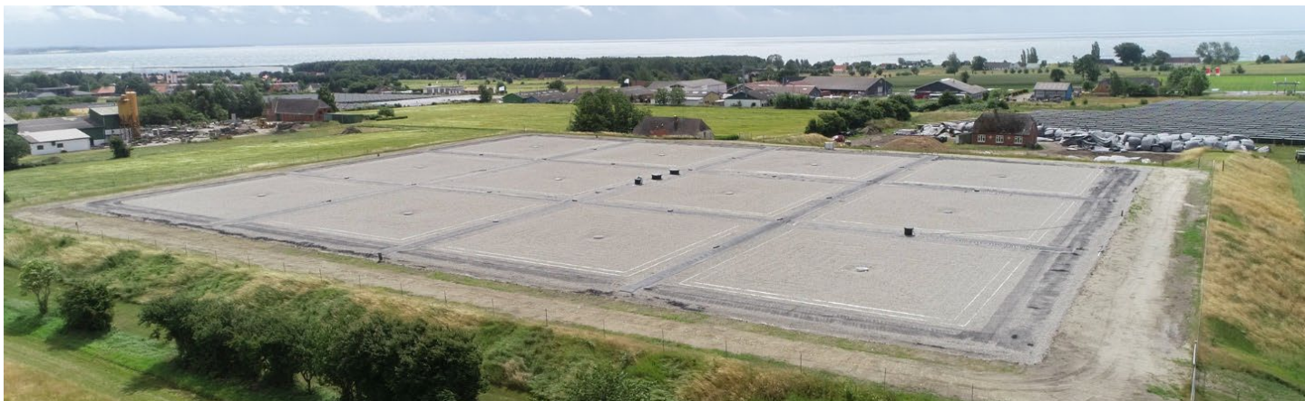
Figure 10. Insulated floating cover on a hot water thermal pit. Marstal, Denmark.
