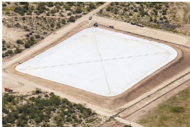
Figure 4. 0.75mm proprietary polyolefin floating cover on a coal seam gas raw water storage to eliminate evaporation, reducing water supply and pumping costs. Texas, USA (Image: Layfield Group)
