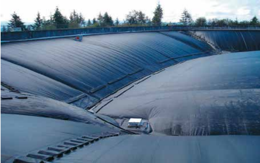
Figure 28. Floating cover being inflated during inspection
