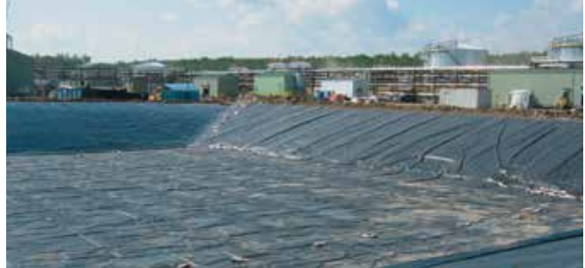
Figure 19. Enviro Liner® 6040 lining a Brine Storage Pond in Ontario, Canada
