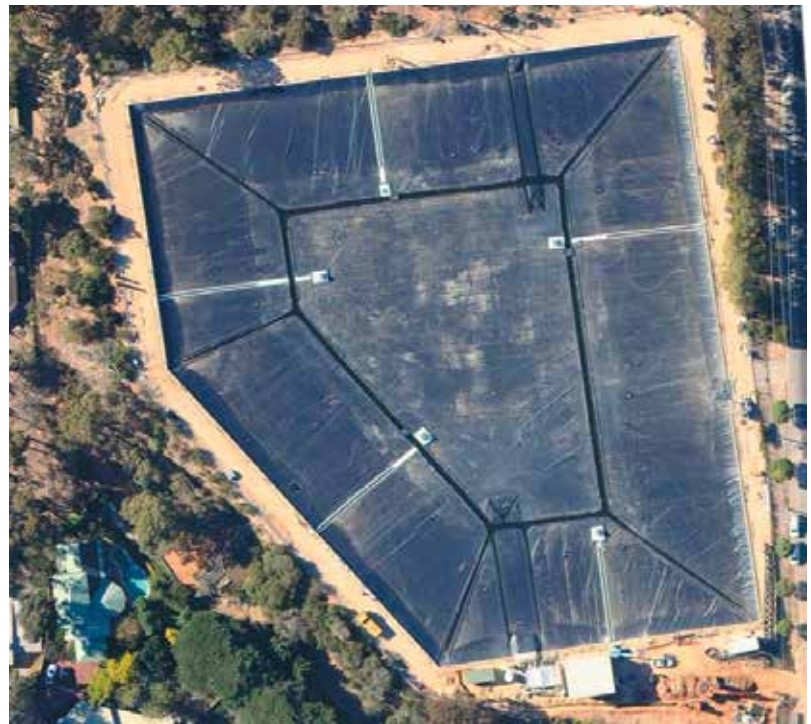
Figure 10. Enviro Liner® 6040 defined sump floating cover for a potable water reservoir in Australia
