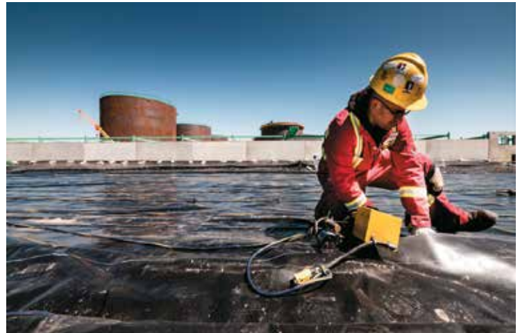
Figure 27. Installation of double lined secondary containment system lined with Enviro Liner ® 6030
