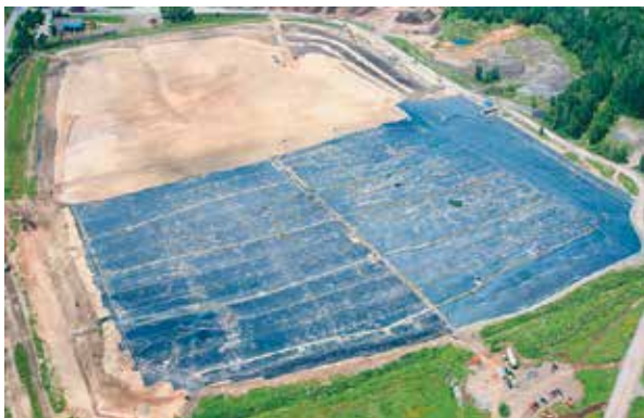
Figure 11. Exposed Landfill cap 3,000,000 ft 2 / 280,000 m 2 Enviro Liner 6030 (30 mil)
