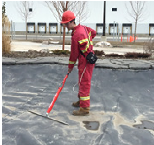
Figure 6. Arc Testing on an exposed geomembrane
