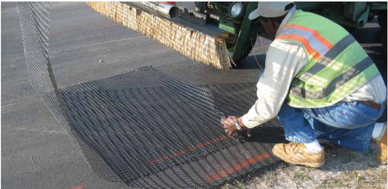
Positioning the GlasGrid product at the transition to a new roll requires some experience and training, however, is easily handled by experienced installers.
