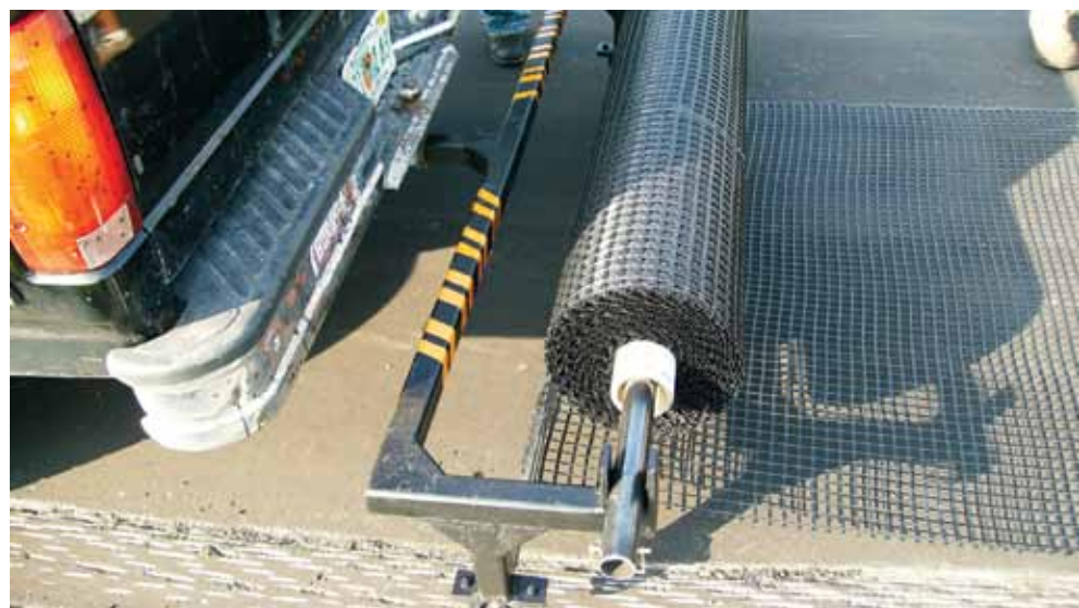
IMAGE J: GlasGrid rolls can be installed manually for smaller pavement areas.
