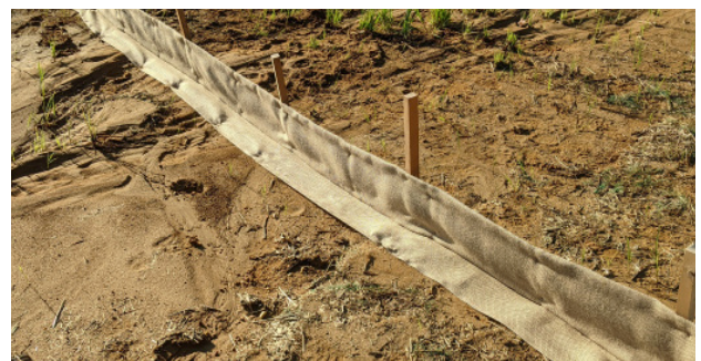
WattleFence Installation, Georgia
