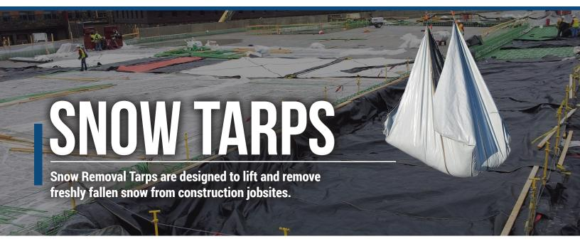
Snow Removal Tarps are used during the winter months to quickly clear the jobsite from snowfall. The tarps are laid out in a grid the day or evening prior to the forecasted snow. They are then simply picked up with an overhead crane or lift after the snow has fallen. Snow Removal Tarps allow contractors to clear jobsites quicker and allow production to move forward. No plowing or shoveling is required, saving valuable time.
