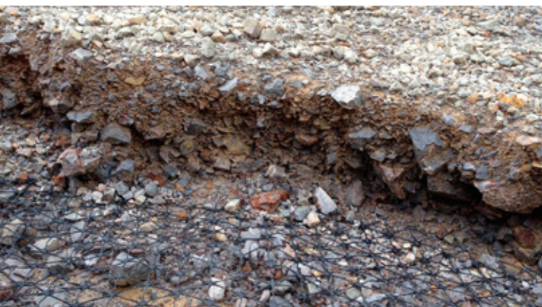
The unique structure of Tensar TriAx Geogrid provides a high degree of in-plane stiffness, improving performance.
