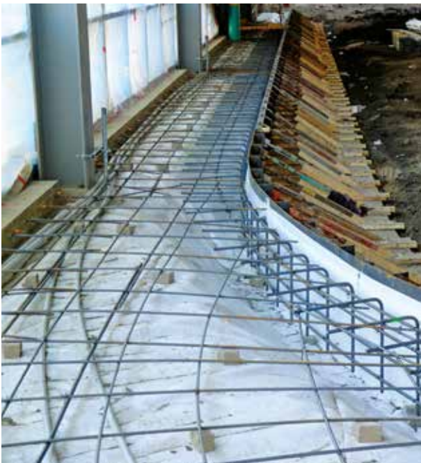
Figure 1. VaporFlex® Standard installation
