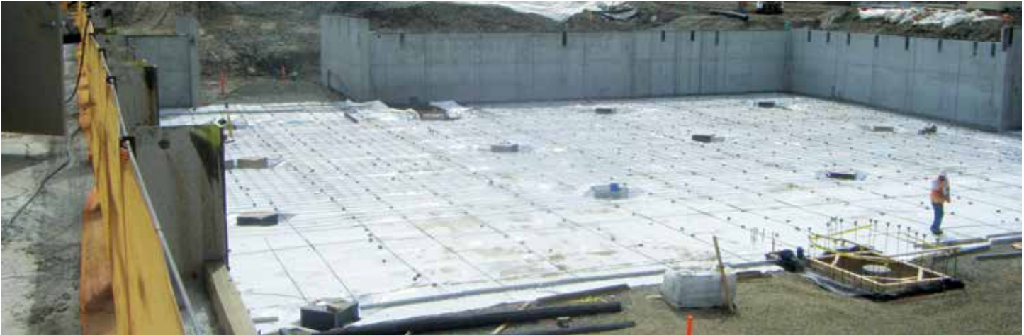
Figure 5. VaporFlex® Standard under building liner application. Swedish Medical Center | Issaquah, WA
