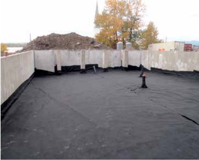
Figure 12. Geomembrane Gas Barrier
