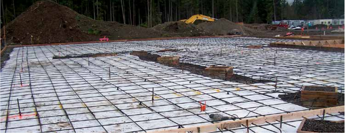
Figure 14. VaporFlex™ Standard underbuilding application.
