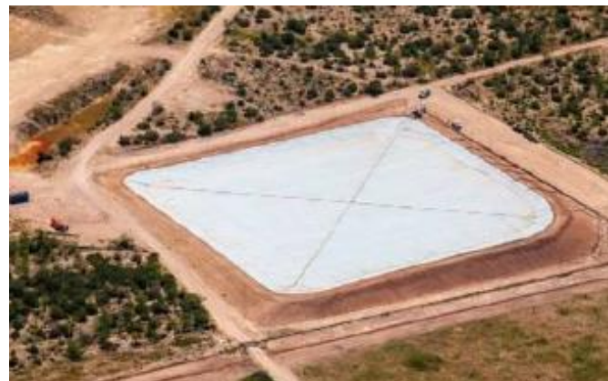
Figure 5. Evaporation Control Cover. Permian Basin, Texas, in 2014
