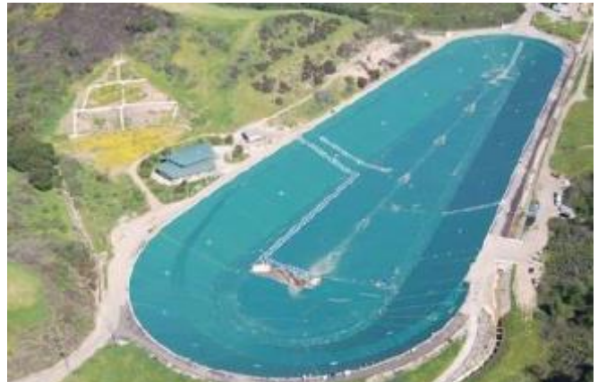
Figure 7. 45 mil CSPE Defined Sump Cover installed in 2019.
