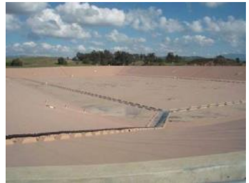
Figure 2. MWDS Skinner Reservoir. CSPE Defined Sump 2013.
