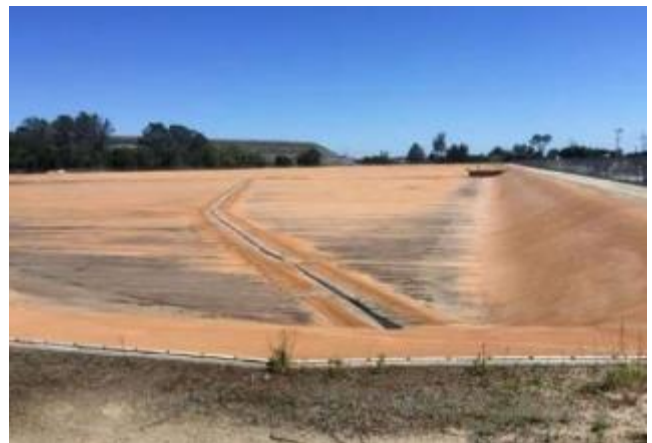
Figure 6. Hinkle Reservoir. 40-year-old cover installed in 1980.
