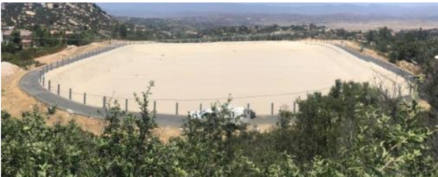
Figure 1. Ramona Water District. CSPE Tensioned Cable Systems installed in 2020.
