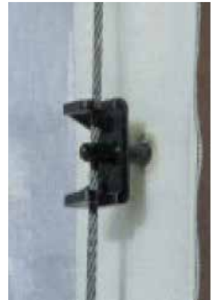
Figure 10. EC 101 and Cable connected to tarp.
